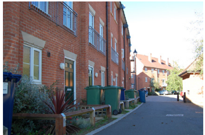
Poorly integrated bin storage erode the quality of this street in Oxford
